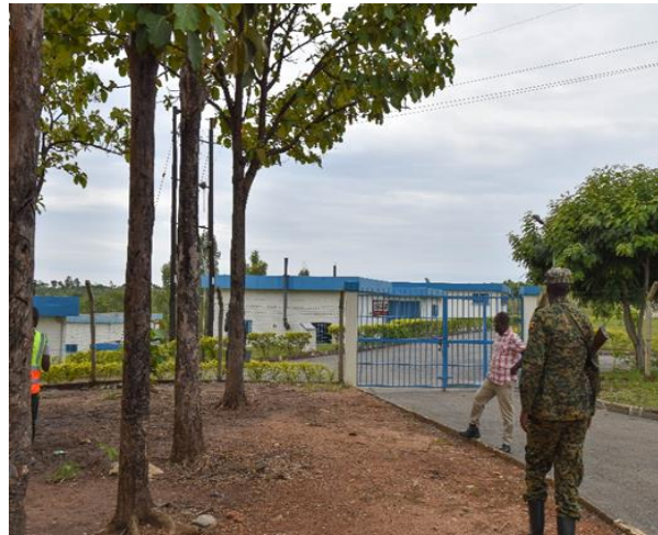
National Water and Ssewerage Cooperation Kochi main treatment plant
